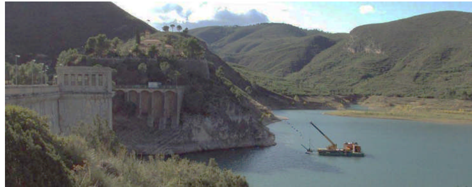
Works in Loriguilla Dam, www.chj.es
