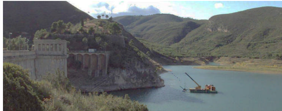
Works in Loriguilla Dam, www.chj.es
