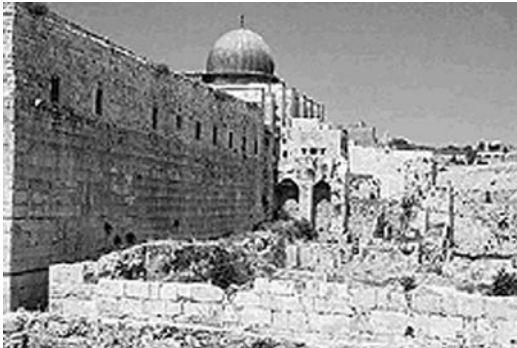
Jerusalem showing water baths and water carrying structures
